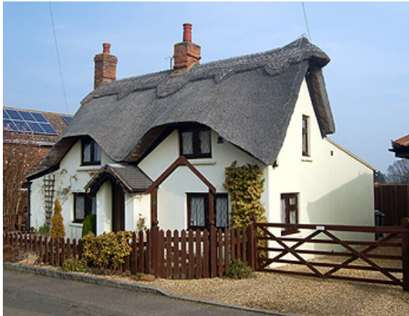
Listed Building Compton Cottage - 12 Ivy Lane
